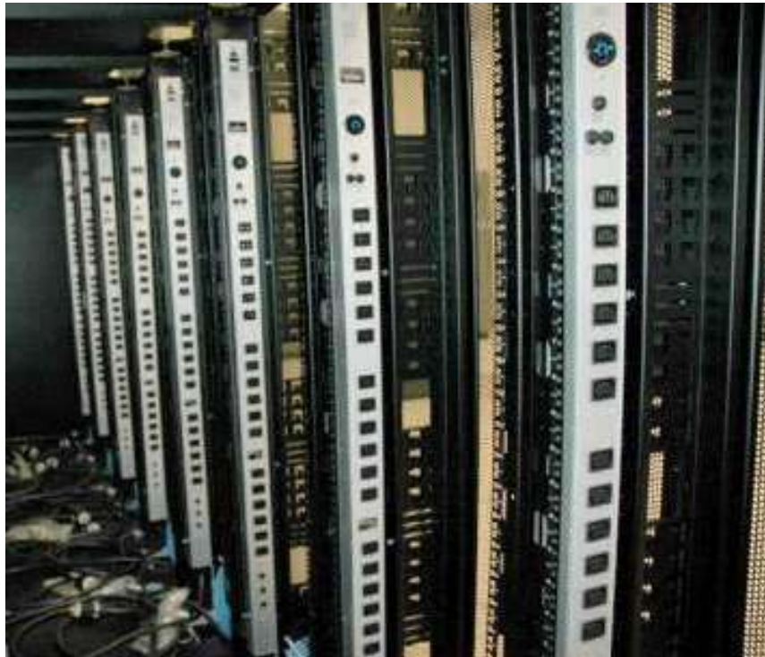
Smart Power Strips Monitor In-rack Power and Environmental Conditions
